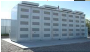
0.8MW Lead Acid Battery 1MW NAS Battery
